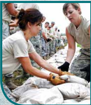
Members of the National Guard lay sandbags to protect against Missouri River flooding.
