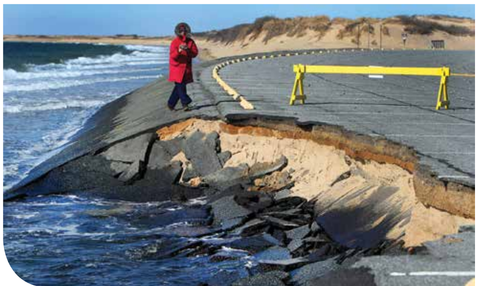
Damage to coastal roads is already a problem along the shores of the U.S. and will worsen as sea level continues to rise.
